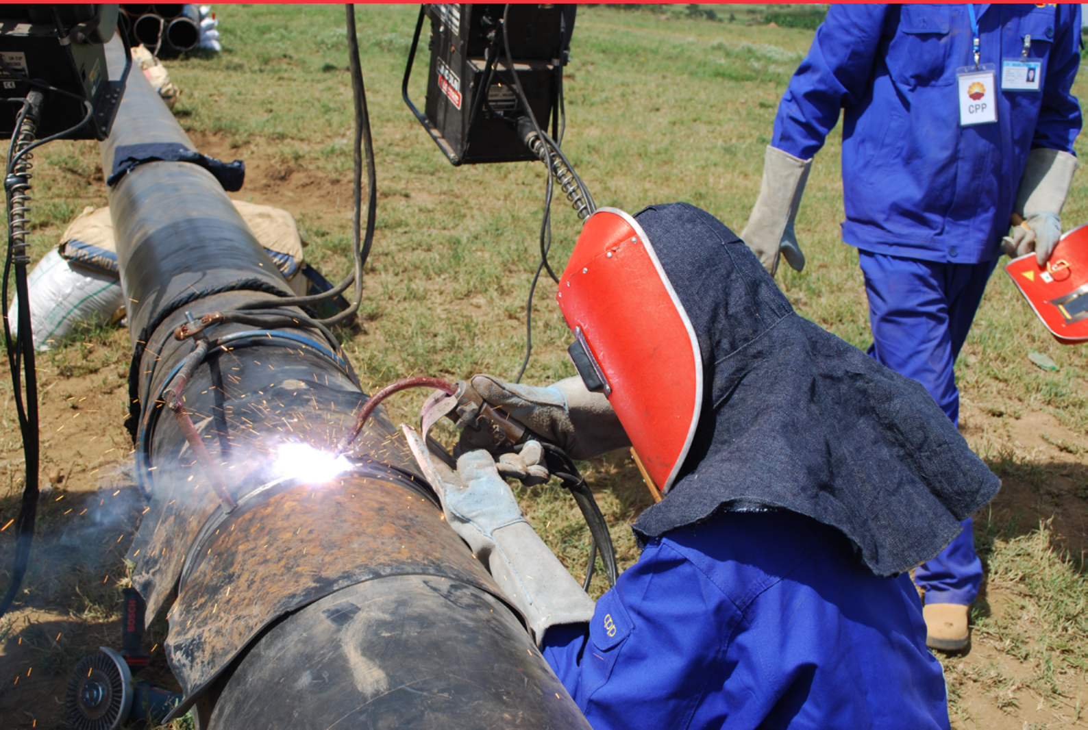
Welding of pipeline
