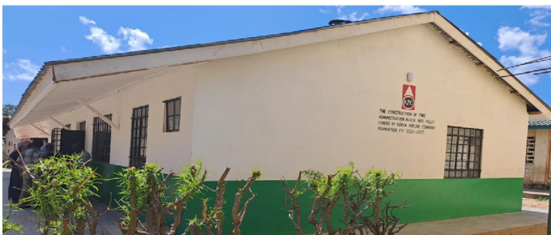
KPC Foundation sponsored the construction of an administration block at a cost of KShs 4 million at Kwahola Primary school in Mombasa County.
