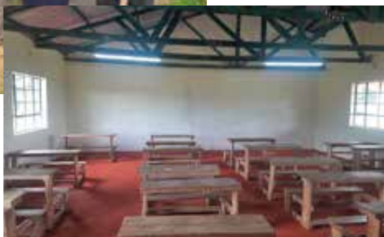
One of the classes that has been constructed in Kamondi Primary School by KPC Foundation.
