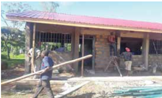
Ongoing construction works at Simbi Secondary School.
